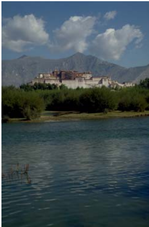
The Potala, seen from across the Lhasa River
